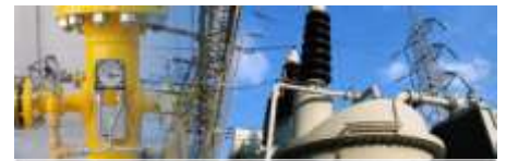
Electric & Gas Utilities
