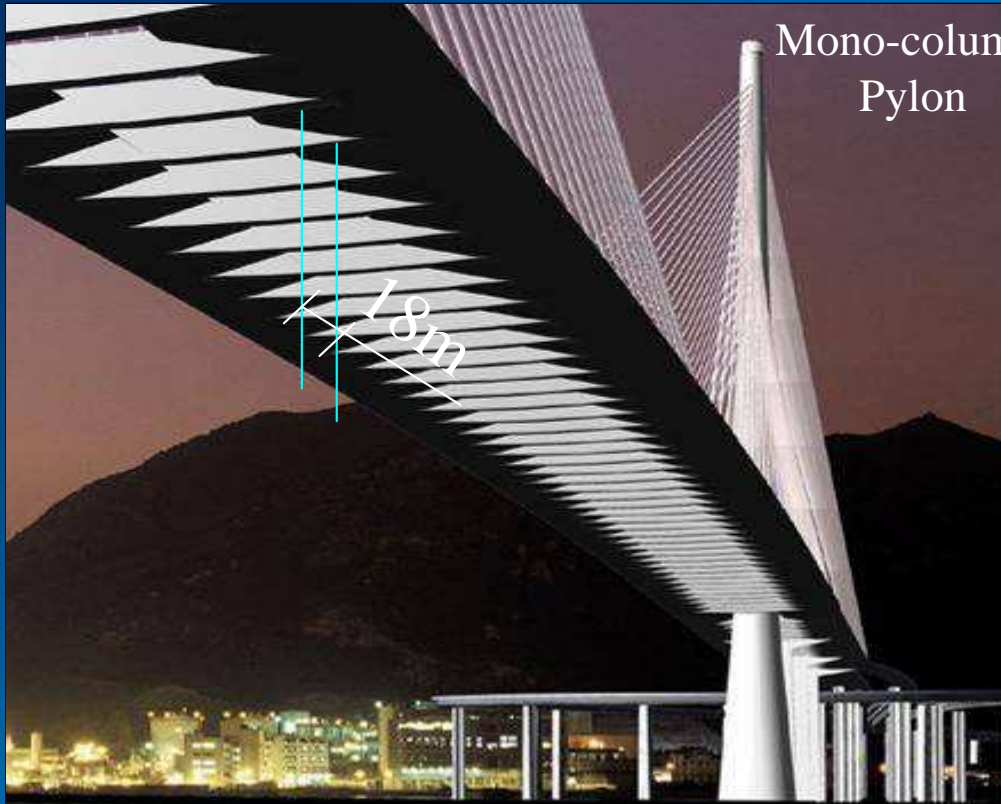
Separated streamlined twin-girder deck
