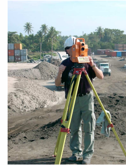
Site setting out
