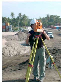
Site setting out
