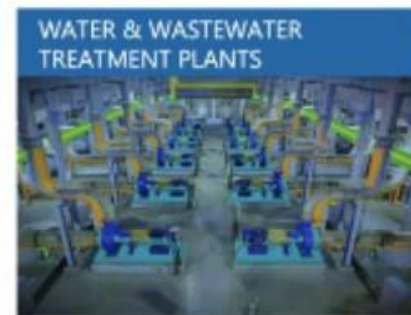
WATER & WASTEWATER TREATMENT PLANTS F. Wayne Hill Water Resources Center Membrane Improvements
