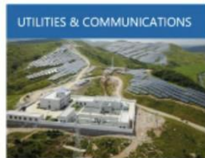
UTILITIES & COMMUNICATIONS Suixian & Guangshui 80MWp Ground-Based Photovoltaic Power Project of Hubei Energy Group PowerChina Hubei Electric Eng. Co., Ltd. China
