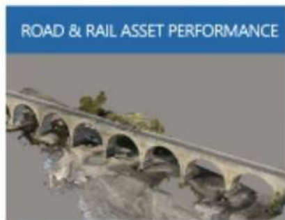
ROAD & RAIL ASSET PERFORMANCE Stone Arch Bridge Rehabilitation
