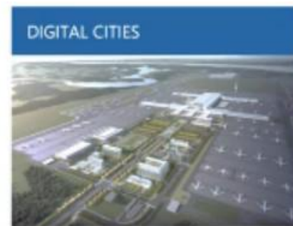
DIGITAL CITIES Ezhou Huahu Airport Project Hubei International Logistics Airport Co., Ltd., Shenzhen S.F. Taisen Holdings (Group) Co., Ltd., Airport Construction Engineering Co., Ltd. China
